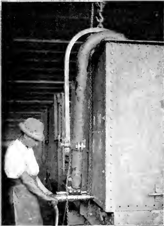
Gap Riveter for Repairing Steel Cars
